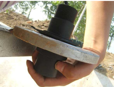
⑦ Screw the nut and fix the transducer
